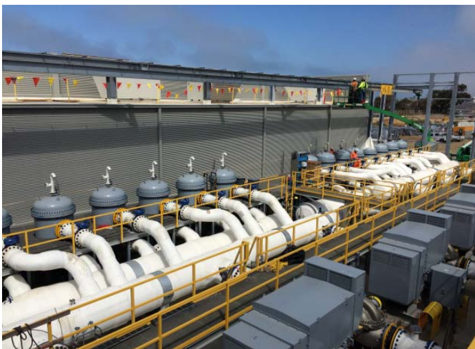
Micro filtration, a pre-treatment ahead of the RO membranes
