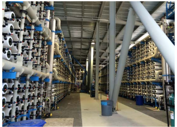
RO desalination membrane banks
