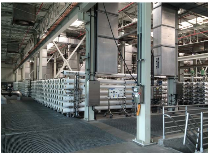
Reverse osmosis membrane banks
