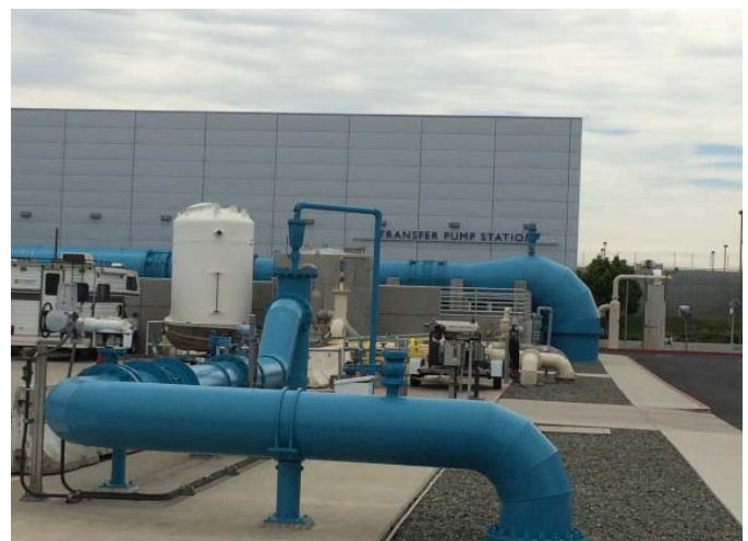
Pump and pipe infrastructure
