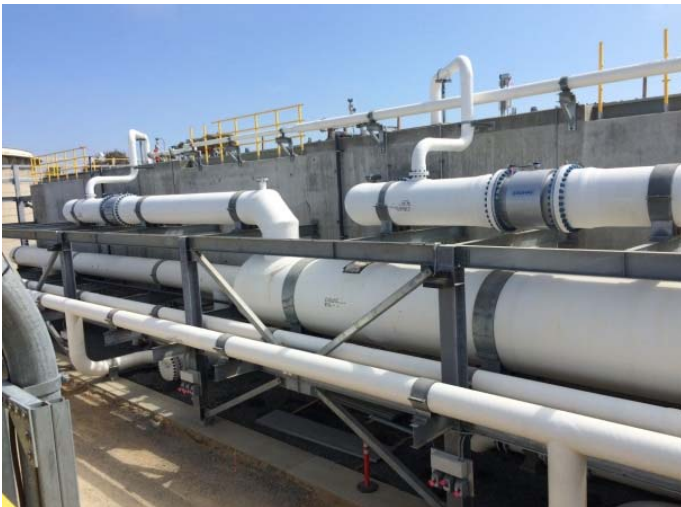
Pipes and pumps move filtered seawater to the clean well
