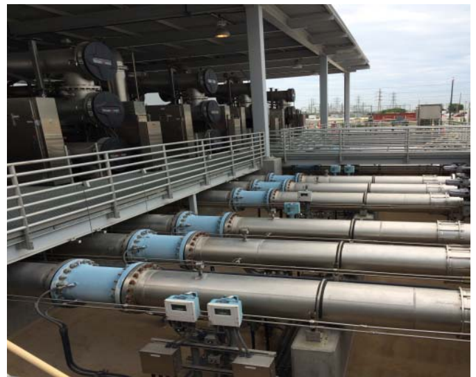
Pipes lead to the UV disinfection units
