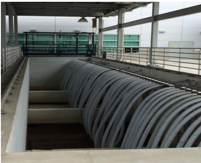
Microfiltration bay at the Orange County Groundwater Replenishment System
