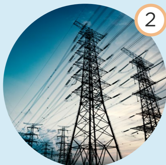
Digital grid infrastructure
